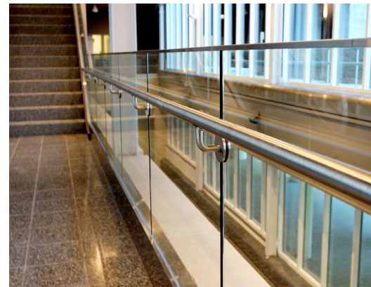
Base shoe glass railing with stainless steel andrail and top cap.
