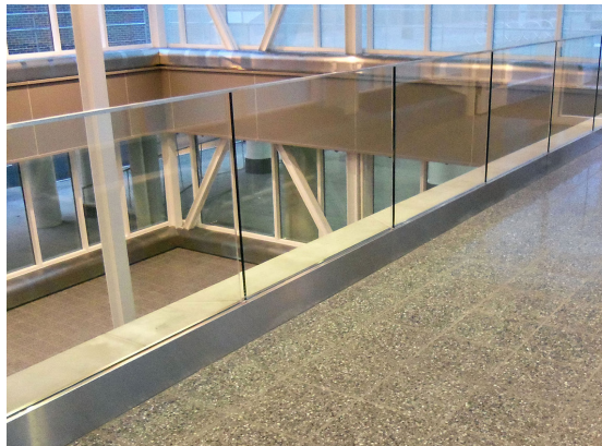
Base shoe glass railing with top cap to minimize deflection.
