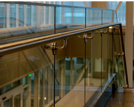
Base shoe glass railing with stainless steel andrail.
