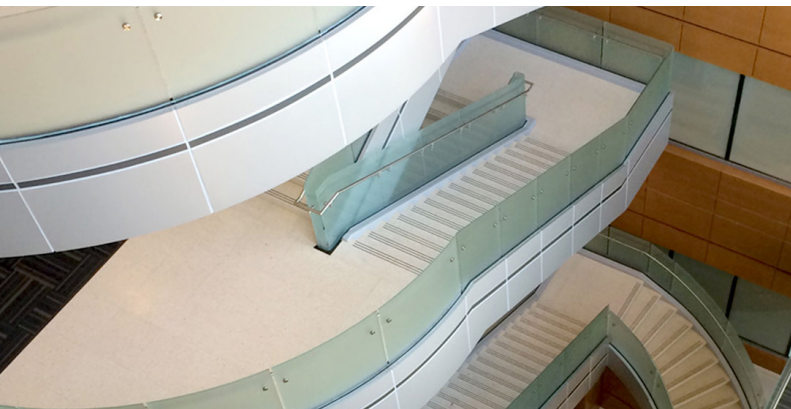
Stainless steel handrails were applied along stairs and landings.
