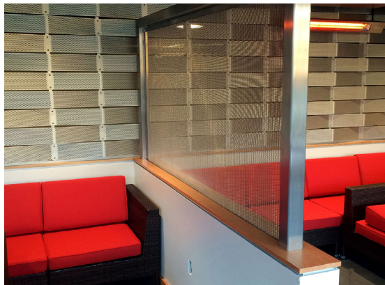
Stainless steel mesh partitions between suite areas.
