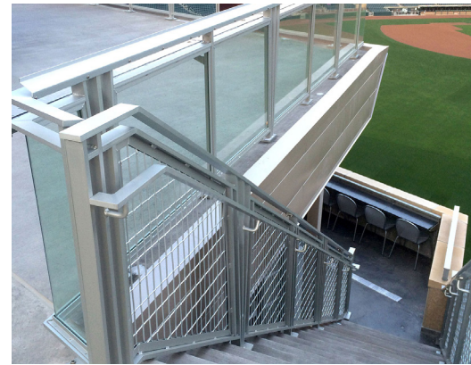
Custom mesh railing on stairs down to "Catch" Suite area.
