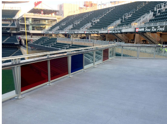
1/2" Optiview clear and colored glass within custom aluminum framed railing.
