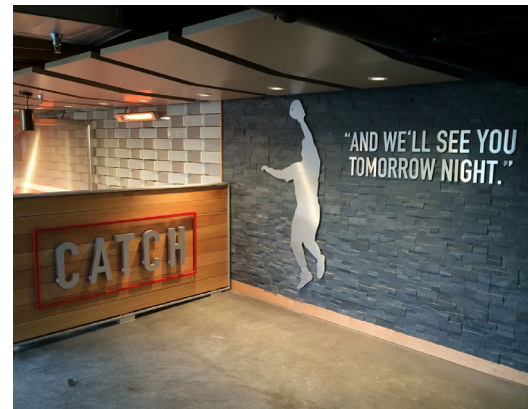
Aluminum framed partition with wood infill leading into the "Catch" suite.
