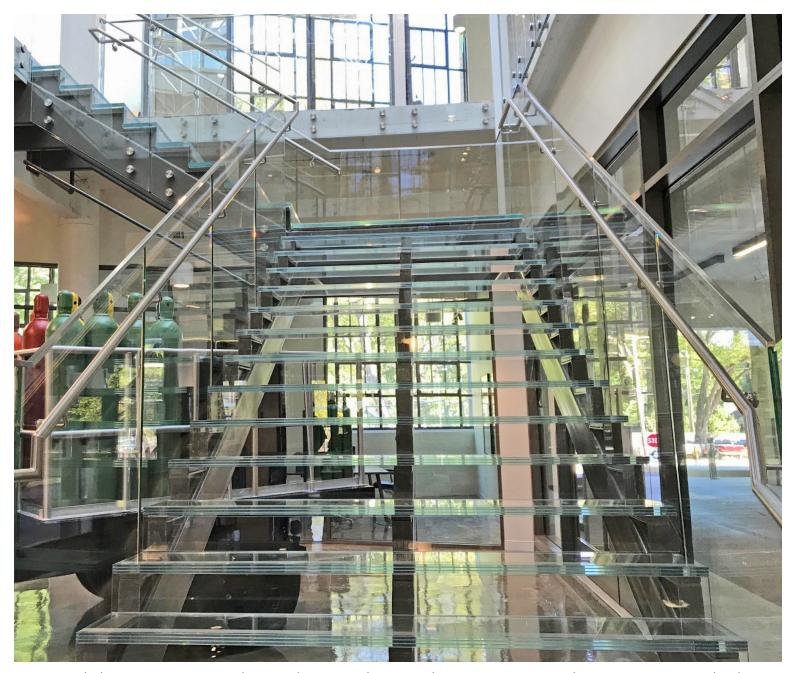
Structural glazing systems are designed in accordance with AAMA, GANA, and ASTM E1300 standards.
