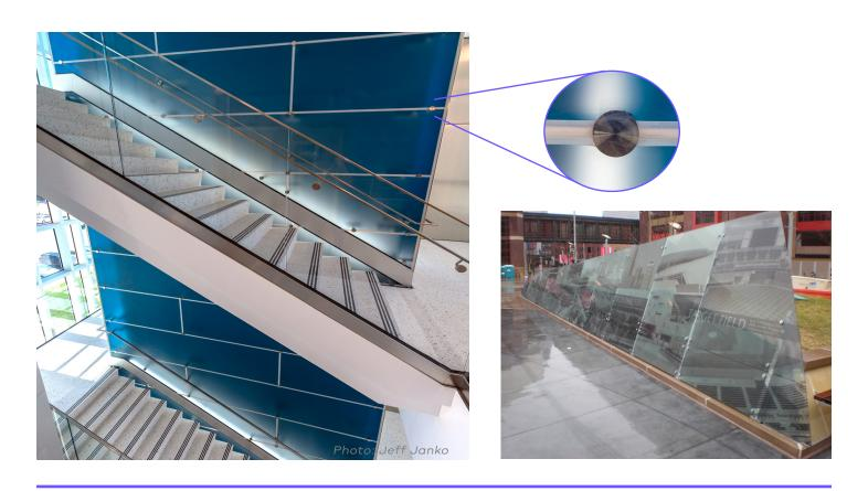
Glass Fins turn traditional glass railing on its edge. Here the glass panels are not only the main structure of the railing, but turning the panels into fins allows for the air flow and more aggressive look compared to standard glass paneling.
