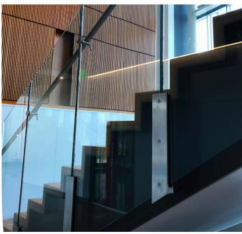
Edge Supported Glass blends the components of traditional curtain walls with railing. The final product is a seamless transition between the two products, allowing the facade to look uniform top to bottom.
