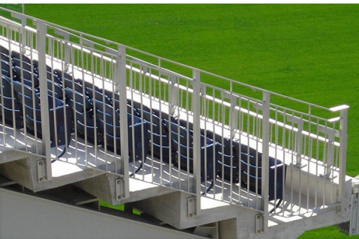
Side mounted Classic Picket Railing with vertical pickets.
