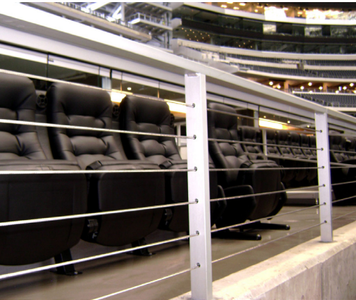
Tensiline cable railing with custom anodized aluminum frame lines the seats to provide an unobstructed view for fans.
