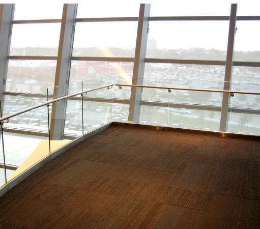
Track Rail base shoe glass railing with 36" high handrail gives a unique view of the skyline.
