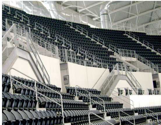
Anodized aluminum aisle railing and Tensiline cable railing throughout facility allows fans to safely get to and from their seats.
