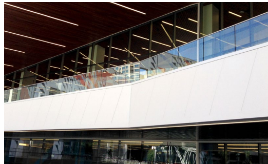
Aluminum clad Base Shoe glass railing with aluminum top cap.
