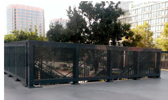
Custom metal railing with aluminum perforated infill panels.
