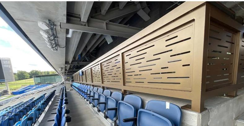
Anodized aluminum finishes in the bowl and brown-bronze powder coating in the back-of-house areas ensure design cohesion and durability.
