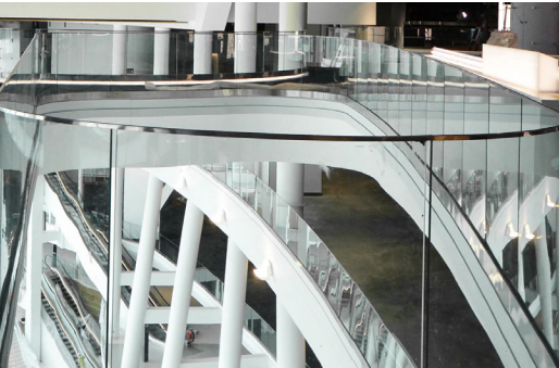
Custom glass railing with curved panels are among the highlights of the arena.
