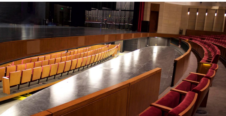
A pit filler platform system was also installed to allow the second row of wagons to become level with the pit area.
