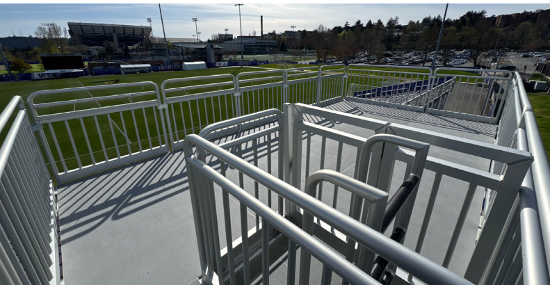
Spanning 30 feet, the system is composed of weather-resistant SC90 Clima-Core platforms and Relia Beam structural framing.
