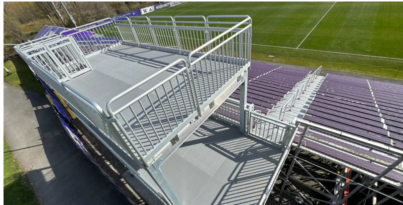
The structure incorporates numerous custom elements, including flip-down railings, cantilevered stairs precisely aligned with the existing stadium aisles and a custom ladder for crew access.
