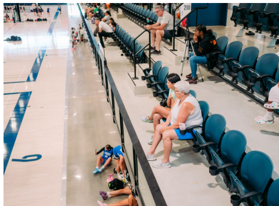
Glass infill panels across seating areas, ensuring both safety and clear visibility throughout the venue's expansive court areas.
