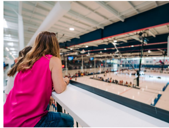
We worked with Turner Construction to engineer drink rails that have the same countertop surfaces used throughout other areas in the building.
