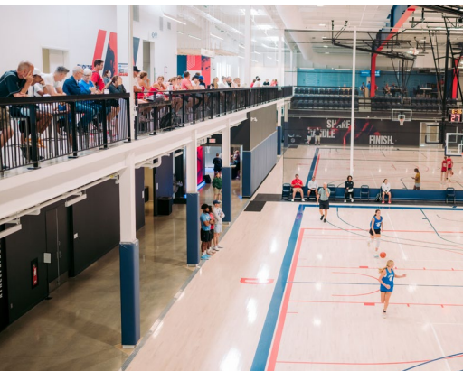
Sightline contributed a wide range of custom-engineered railing systems totaling nearly 2,000 linear feet.
