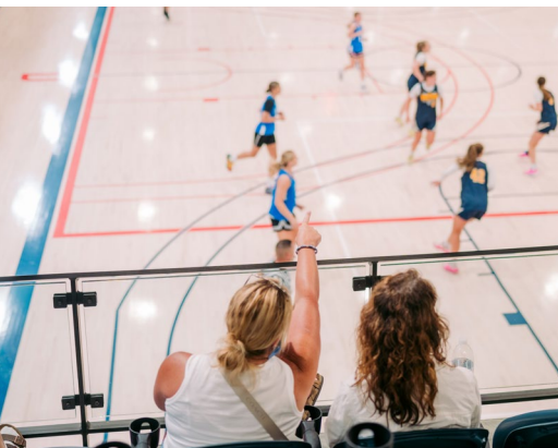
We coordinated installation of railing with 9/16" glass infill with a PVB interlayer along the front of the spectator bowl.
