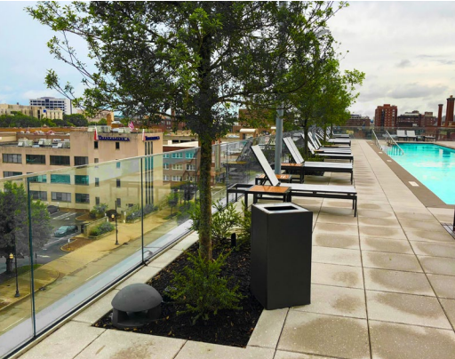
To optimize views, custom SGP laminated glass guardrail surrounds the rooftop pool on the third floor.
