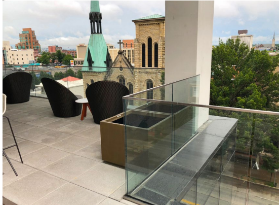
The exterior glass guardrail that lines the rooftop pool area provides an enjoyable environment and outdoor experience.
