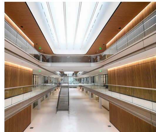
2,500 linear feet of Track Rail was designed for PGA TOUR's new Global Home.
