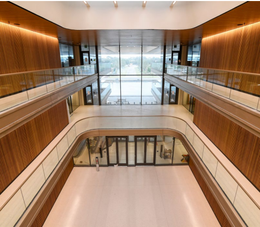
Clear 9/16" laminated glass railing offers unobstructed views and adds a luxurious accent to the 44' tall Grand Atrium.
