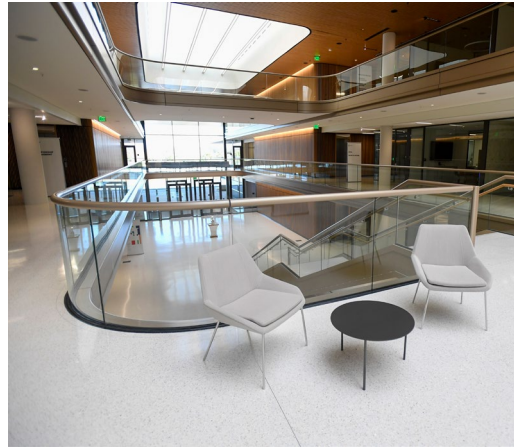
Nearly 300 linear feet of curved glass Track Rail with custom-extruded aluminum top cap can be found throughout the atrium.
