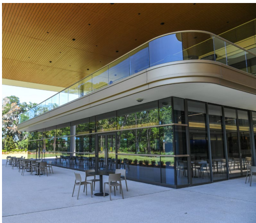
Track Rail extends to the exterior balconies, optimizing views of the lush natural surroundings.
