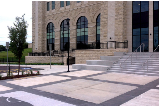
Custom steel guardrail lining entrance to facility.
