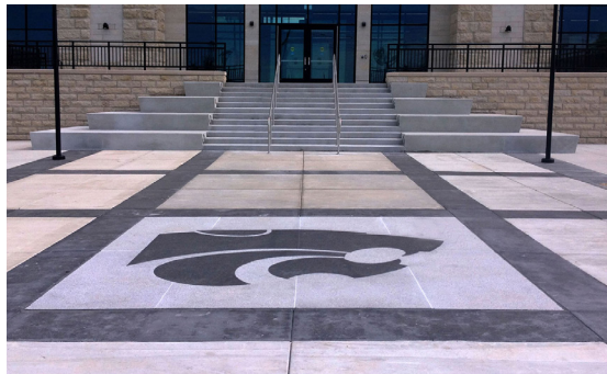
Custom steel picket style guardrail.
