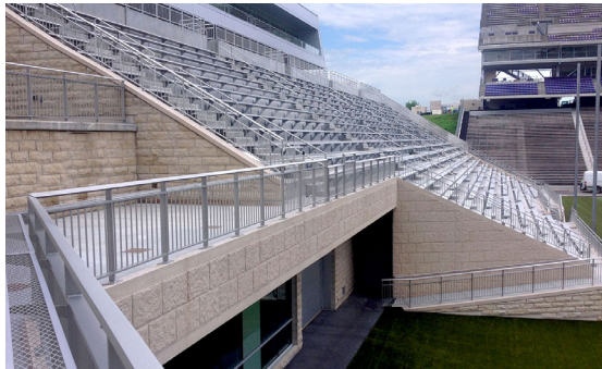
Wabash Landing showcasing aluminum picket railing with custom mesh drink rail.
