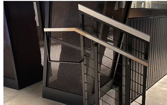
Aluminum picket style railing at front of ADA areas.
