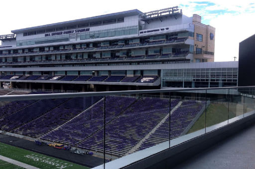
Balcony overlooks utilize Base Shoe railing with aluminum top cap and 1/2" glass infill.
