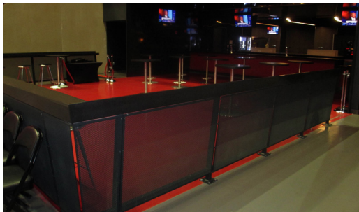
Custom railing system with aluminum perforated panel infills.
