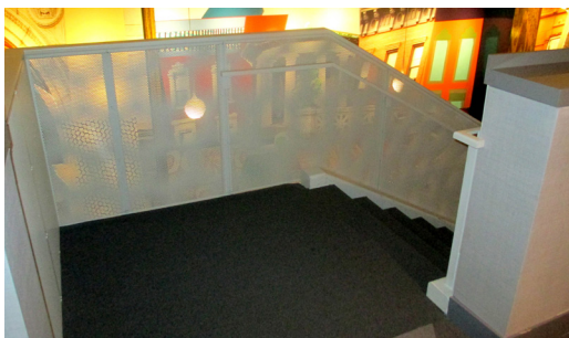
Custom railing system with aluminum perforated panel infills.
