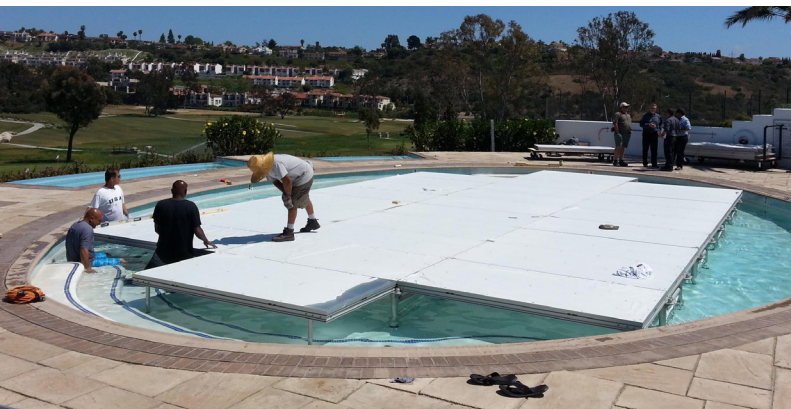
Sightline engineered a custom pool cover using acrylic platforms and SC9600 bridge supports to create additional surface area.
