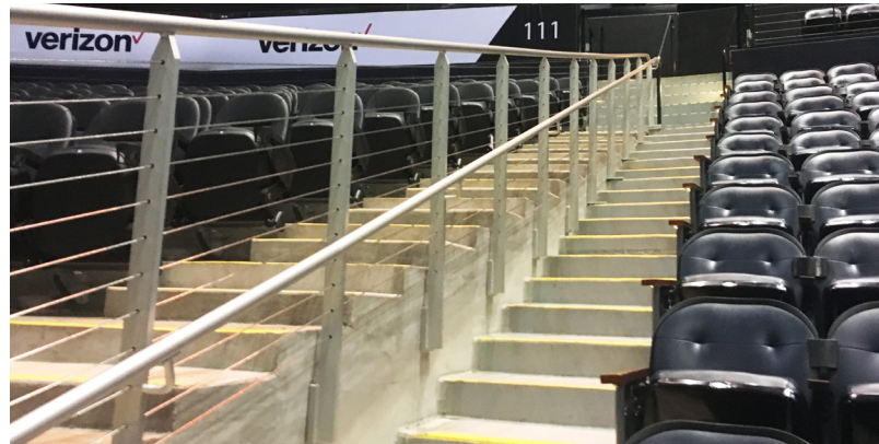
A combination of Tensiline Cable Railing, Griprail and Classic Picket Railing can be found throughout the arena.
