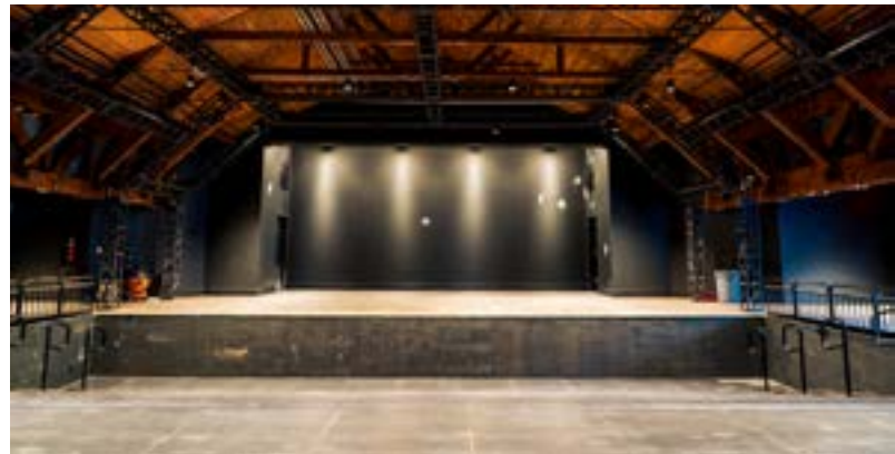
This project required four SC90 riser sections, a full stage trap system and IBC-compliant railings and sockets.
