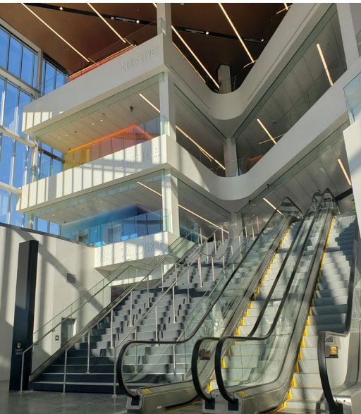
For improved crowd access, the renovated lobby boasts new elevators, escalators and monumental stairs lined with Sightline glass guardrail.
