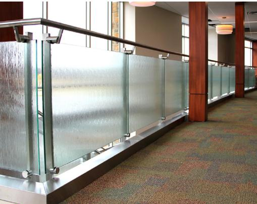
Dot series railing system with handrail at 42".
